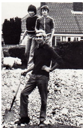
Russ working on the embankment in 1978
