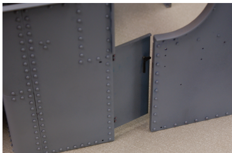
Cab doors now fitted to the 15XX
